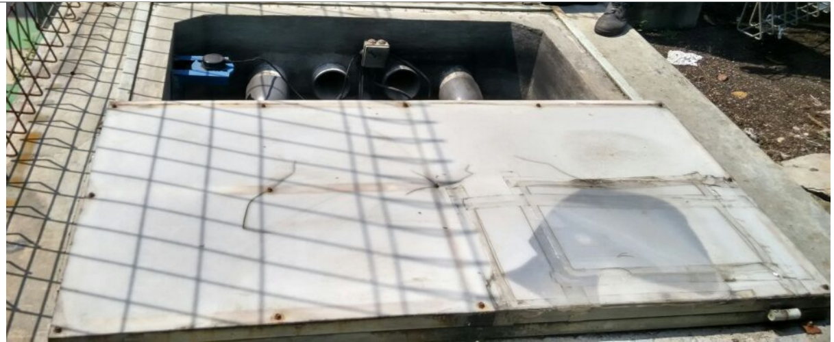
We installed a rainwater harvesting unit at our Indonesia manufacturing facility.
