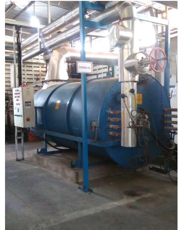
Energy-efficient heater installed at our Susemi manufacturing unit in Indonesia
